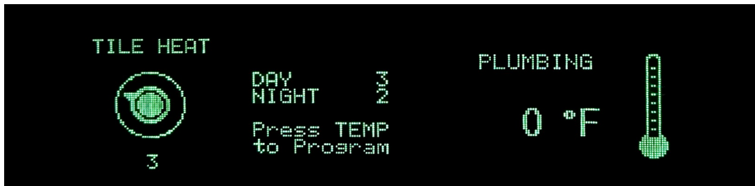
Tile Heat Status Screen
